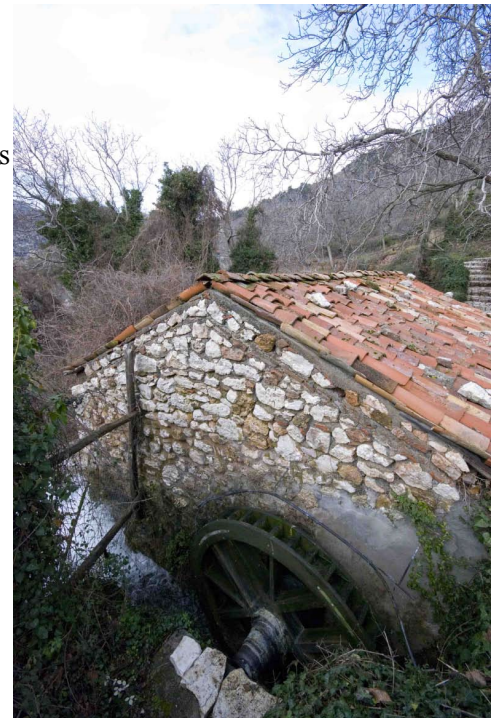
The upright wheel of the gunpowder mill
