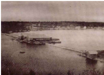
Morse Dam– Winnegance in background (Photo: MMM)
