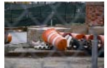
Millstones during construction - they are in the box the millstones within the construction site before the community outcry moved them.
