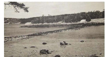
Remains of the dam – about 1954 (Photo – Peabody)
