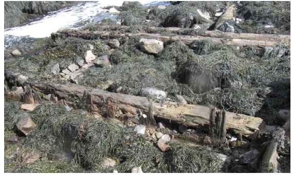
Pond-side sheathing, Bell Mill Edmunds ME is supported by sill timber.
