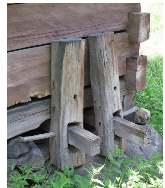
02 The fixing of the hammers
