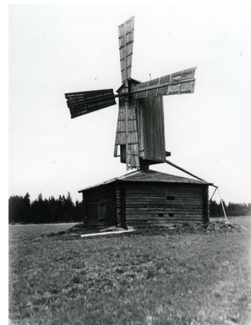
So-called magpie mill (hollow post mill) at Punkalaidun, Satakunta region (coll. The Mills Archive, Reading, UK)
