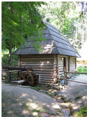
25 A flour mill with small overshot wheel
