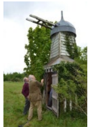
Figs. 8 & 9. The cap, and Dave Pearce operating the brake lever.
