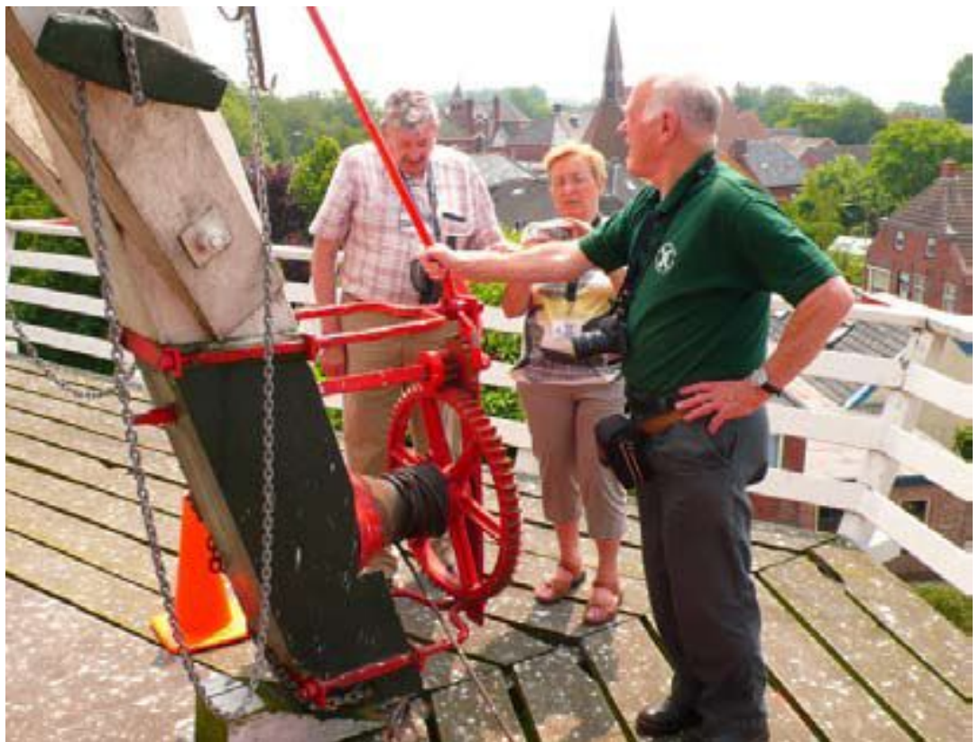
Most windmills in The Netherlands are tail winders. Here we see participants studying and discussing the regional variations of the winding mechanism.
