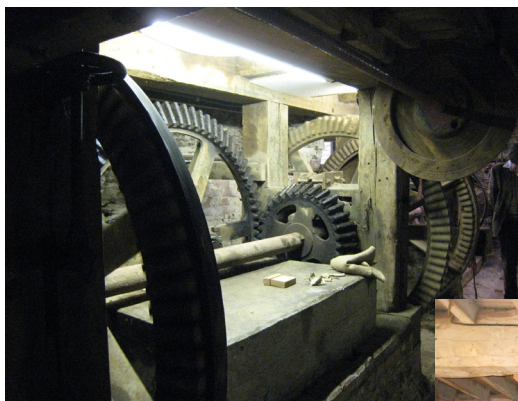
Unusual lay shaft gearing at Bridgetown Water Mill
