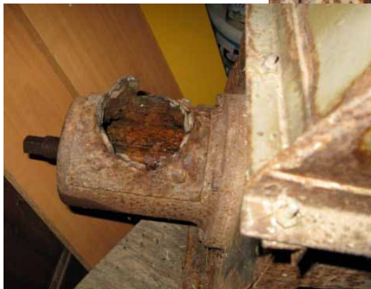
The entry point for the water turning the water wheel
