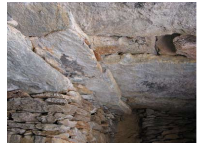
The hole in the stone roof to allow the fumes to escape.
