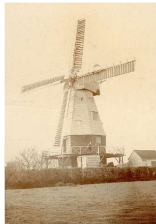
Benenden windmill, Kent 1910, showing wooden windshaft and men on reefing stage
