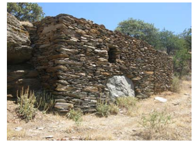
The oil mill with an old flat stone in the wall. One can see the wall built against the cliff to enlarge the cave.
