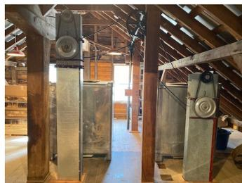
*Third floor elevator heads. Water powered hopper, bottom grain bins in background.*
