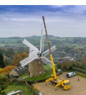
last of the 42 old shutters, which had been fully refurbished, was put in place. Some pieces of the heavy iron work which operate the shutters, taken from the old sails, were re-fitted and the job was virtually done.
