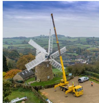
20th September, the last of the 42 old shutters, which had been fully refurbished, was put in place. Some pieces of the heavy iron work which operate the shutters, taken from the old sails, were re-fitted and the job was virtually done.
