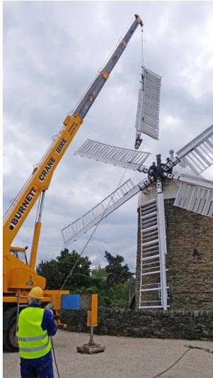
*The last of the sails is lowered into place by the mobile crane.*
