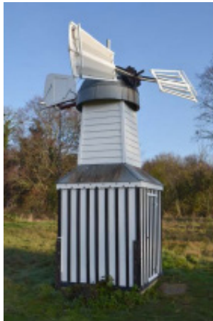
The mill, complete with new boards, door, rudder and two sails (December 2020).
