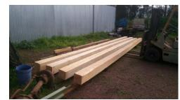
Spruce beams 200mm square and 8m long are in my yard for use as stretchers, braces and tail-pole.
