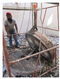
Friends of Mostert's Mill reacted quickly. All the metal pieces were collected and put away. The millstones are re-useable although the bed-stone is cracked.
