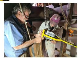
The upper brake assembly is more than half a circle so we could measure the diameter, and we stopped cutting when we had about 5mm clearance.
