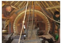
We tried the upper brake assembly but it wouldn't fit, so we decided to machine it to fit exactly, using my router suspended from a central point. We measured the new circumference and calculated the radius.
