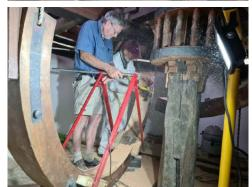
The router is suspended from a pipe which is supported by two A-frames, bolted to spacers which were screwed to the brake blocks. The spacers allowed the centre of the router to reach the outer edges of the brake blocks.
