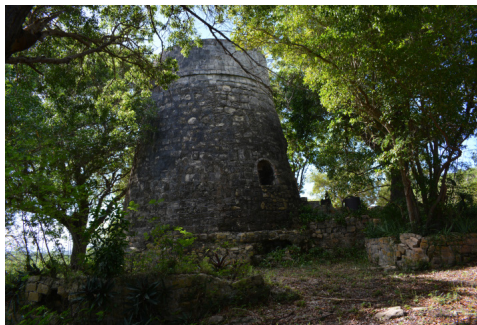
Fig. 6 The juice trough opening facing the camera here was completely blocked up and the bottom portion of the bagasse opening to the right was blocked up, likely when the estate Sion Hill windmill was still in operation, and this may have indicated a shift to crushing cane outside the tower with horizontal crushing machinery
