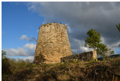
Fig. 4 The windmill at estate Windsor and Windsor Forest was converted to a cistern to store water after decommissioning.
