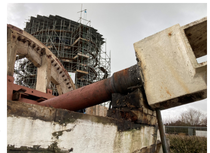
Fig. 3 Detail of break wheel and canister block 2026. Image credit: Mark Rickards
