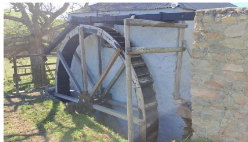
The new launder Thys had made, with sloping extension to minimise splash.
