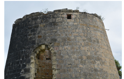
Fig. 15 The small square near the top of the Paradise and Downings windmill is the exit of the flue. For some reason, most of the internal chimneys go between the top of the machine slot and the top of the mill.
