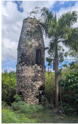
Fig. 30 Windpump, pump mill, well tower at estate Little Princess , where the water level is nearly at ground level
