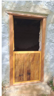
Smart new old-Yellowwood door installed.
