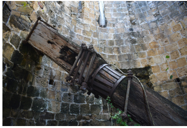
Fig. 7 The windshaft at the Bonne Esperance mill
