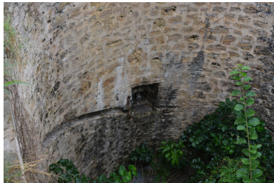
Fig. 11 Each of the windmills at Castle Coakley has a large masonry-lined area beneath the mill to remove the crushed cane bagasse from the mill by donkey cart. In this image, the slanting channel on the left goes down to access one of the cisterns in which cane juice was collected.
