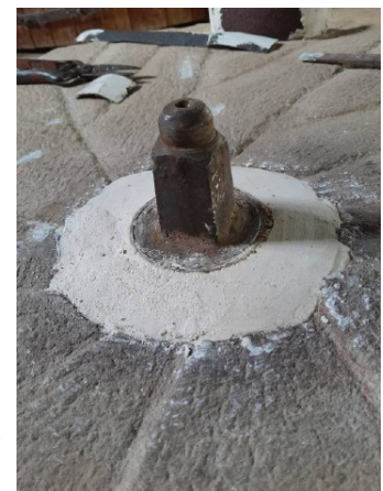
Plaster of Paris cone at the top of the neck bearing.
