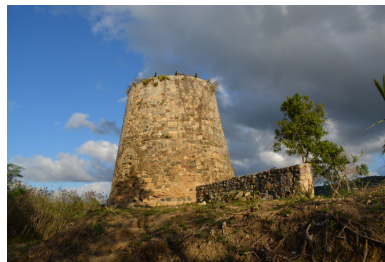
Fig. 4 The windmill at estate Windsor and Windsor Forest was converted to a cistern to store water after decommissioning.
