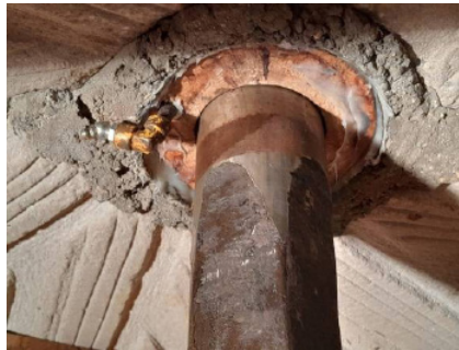
The underside of the neck bearing fixed in place with Epidermix.
