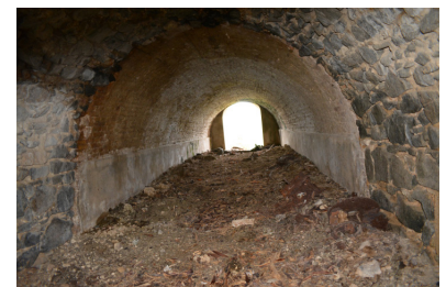
Fig. 13 The main basement at The Sight windmill is over 5 feet high and runs the full width of the windmill
