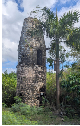
Fig. 30 Windpump, pump mill, well tower at estate Little Princess , where the water level is nearly at ground level
