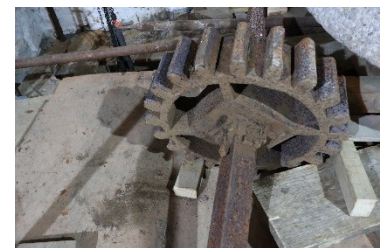
Shaft bearing and gear
