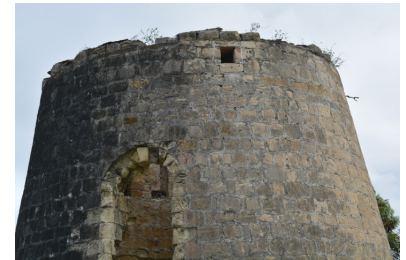
Fig. 15 The small square near the top of the Paradise and Downings windmill is the exit of the flue. For some reason, most of the internal chimneys go between the top of the machine slot and the top of the mill.
