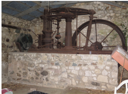
Fig. 21 Steam engine at estate Rust op Twist
