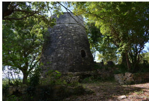
Fig. 6 The juice trough opening facing the camera here was completely blocked up and the bottom portion of the bagasse opening to the right was blocked up, likely when the estate Sion Hill windmill was still in operation, and this may have indicated a shift to crushing cane outside the tower with horizontal crushing machinery
