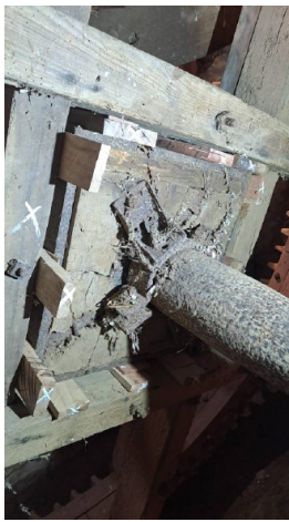
Three pairs of folding wedges on each face.
