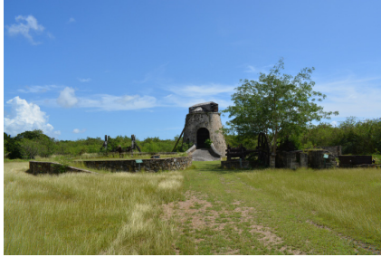
Fig. 24 At The Whim, the animal mill is on the left, the windmill at the center, and the steam mill to the right. All fed the boiling house on the far right.
