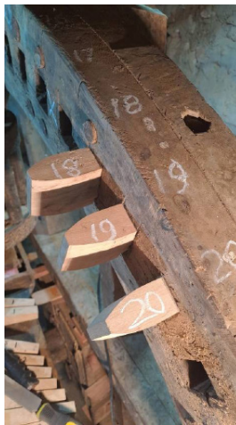
Fitting new cogs to the sockets. I was showing Thys how stiffly they should fit.
