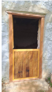
Smart new old-Yellowwood door installed.
