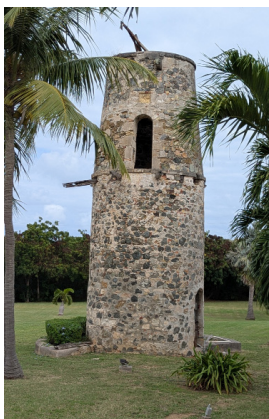
Fig. 28 Windpump, pump mill, well tower at estate Mount Roepstorff and Southgate Farm
