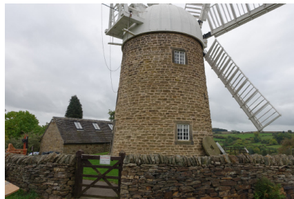
Fig. 1. The mill after all the lime pointing has been completed
