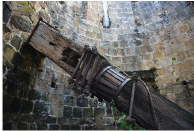
Fig. 7 The windshaft at the Bonne Esperance mill
