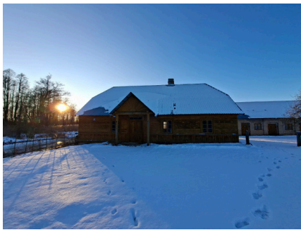
Main silhouette of the mill building with the front door; the household had a side entrance on the north
