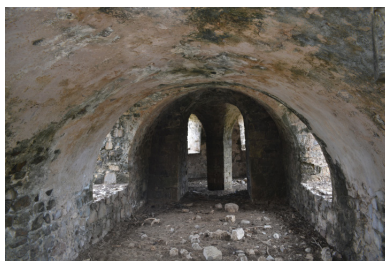
Fig. 12 Looking down the length of the basement under the access ramp to the mill above, with the distant central pillar supporting the working floor of the Diamond Keturah windmill
